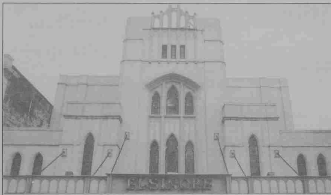
The Elsinore facade is adorned with lots of stained glass which is in need of expensive repairs.
