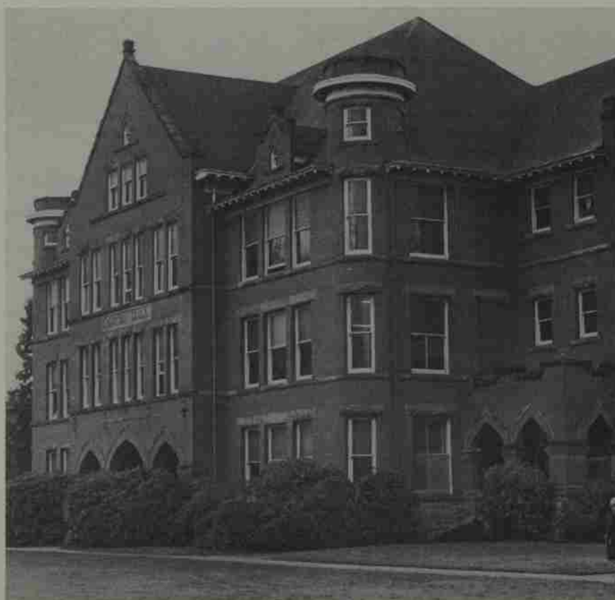
Eaton Hall is the second phase of the Campaign for Willamette and renovation work began in mid-July on the $1.7 million project. The building, a Salem landmark, will undergo remodeling throughout the interior and will be ready for use in January when Willamette's spring semester begins. The new campus mail center and several administrative offices formerly in Eaton are now housed on the first floor of the Putnam University Center where further remodeling has taken place to accommodate the switch.
