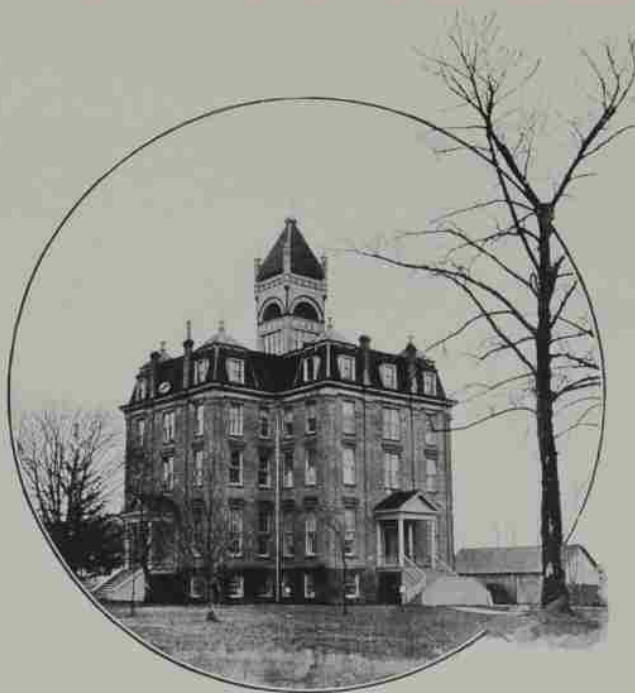
New roof after the fire of 1891.
