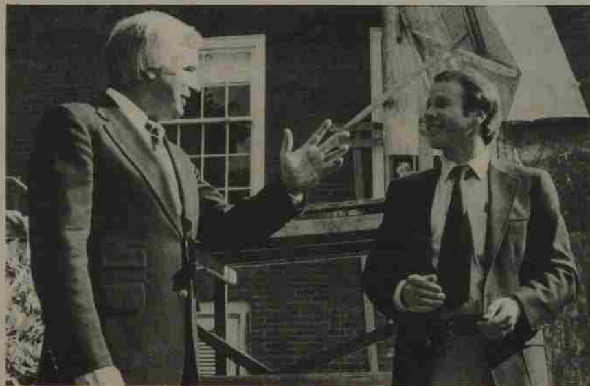
New president Dr. Jerry Hudson, left, discusses Willamette's future with Vice President for University Relations, Larry Large, as renovation of Collins Hall continues in the background.
