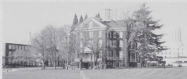
1992—Waller Hall was the subject of a commemorative stamp celebrating historic buildings of the U.S.
