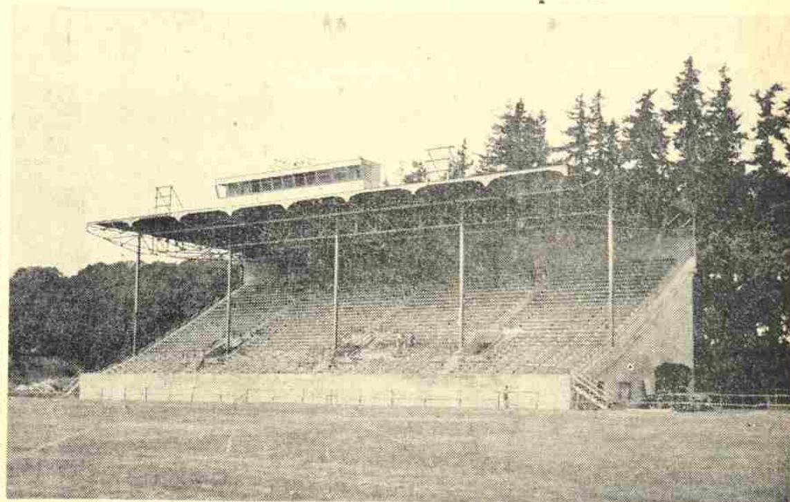
Pictured here in a still uncompleted state is McCulloch Stadium, the $200,000 project at Bush's Pasture. Willamette and CWCE will initiate the new stadium when they square off for the first grid battle of the season tomorrow afternoon at 2 p.m. The stadium will be dedicated on October 14 when the Bearcats meet the University of Hawaii.
