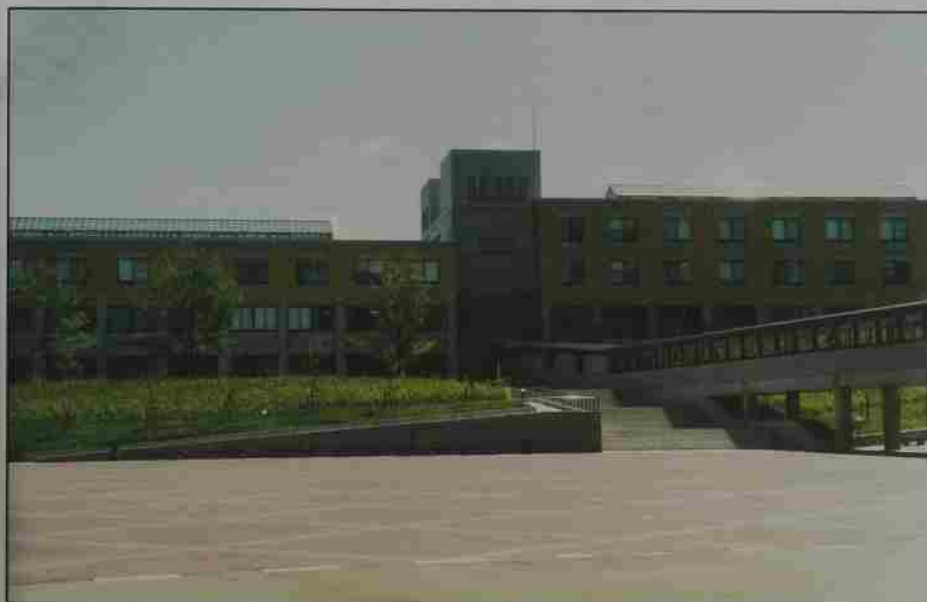
Aomori Public College. A view of the south wing with the bridge which connects the classroom area to the gymnasium. Deep winter snows make students and faculty appreciate the bridge.
