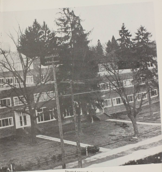
Situated among the trees on the northeast corner of Willamette campus is the new men's dormitory, Baxter Hall. Completed in time for use the second semester, the hall houses the independent and four fraternity wings. Baxter accommodates 224 men and was constructed under the watchful eye of awe-struck students. A beautiful building, the hall has all the most modern furnishings and conveniences and those living there are greatly envied.
