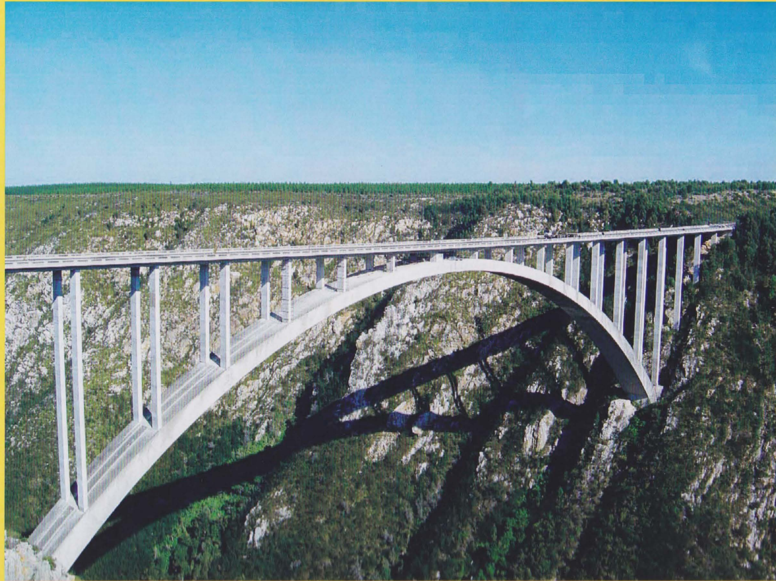
The Storms River Bridge, home to the highest commercial bungee jump in the world, 219 meters.
