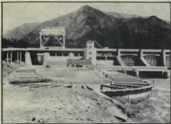
Fish Ladder At Bonneville To Allow Salmon To Reach Spawning Beds
