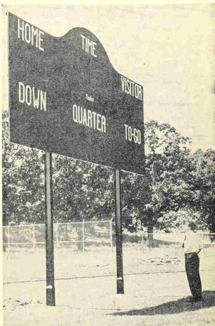
This large new electric scoreboard, erected by the Tidewater Associated Oil Company, will greet football followers at McCulloch stadium this season. Looking over the fully equipped board is Jim Finney of Portland, construction engineer for the oil company. The welcome addition to the stadium is at the south end of the playing field. (Cut courtesy Oregon Statesman.)
