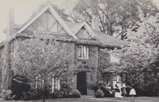
Chi Omega House — 425 N. 14th Street
