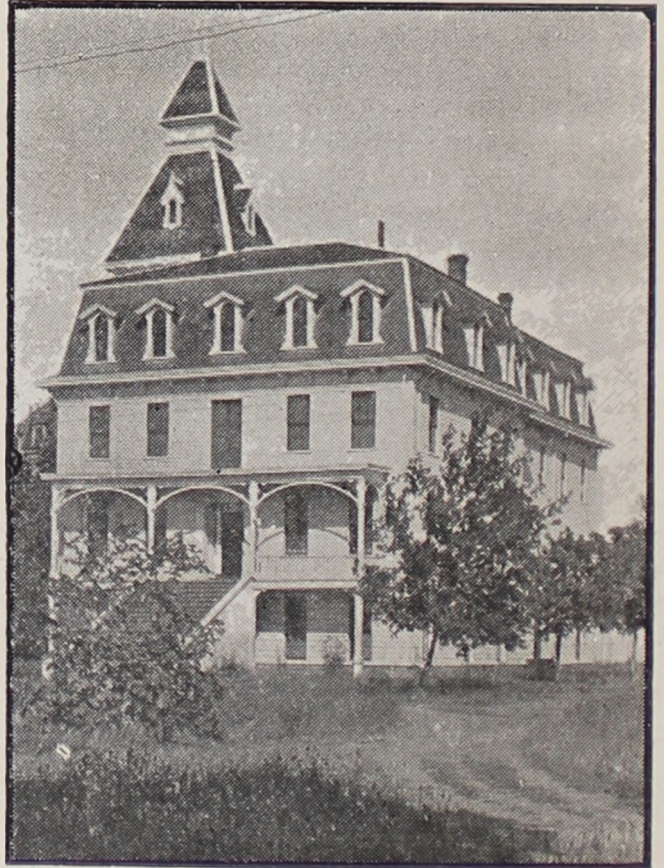
Lausanne Hall—Ladies' Dormitory.
