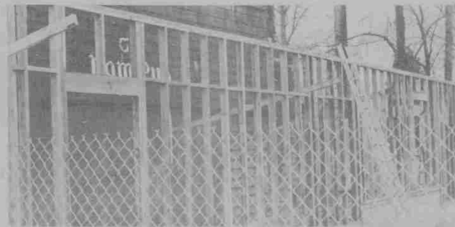
The Ram Pub in the beginning stage of remodeling.
