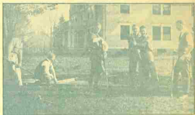
Typical Scene in Construction of New Walk.
