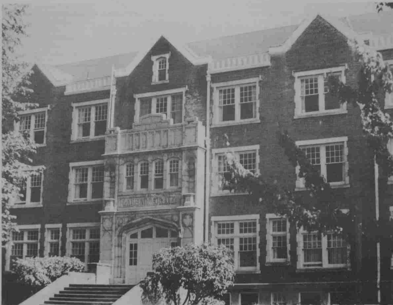
The University was recently denied a federal housing loan to renovate Lausanne Hall, long considered a fire hazard. photo by Barb Herr
