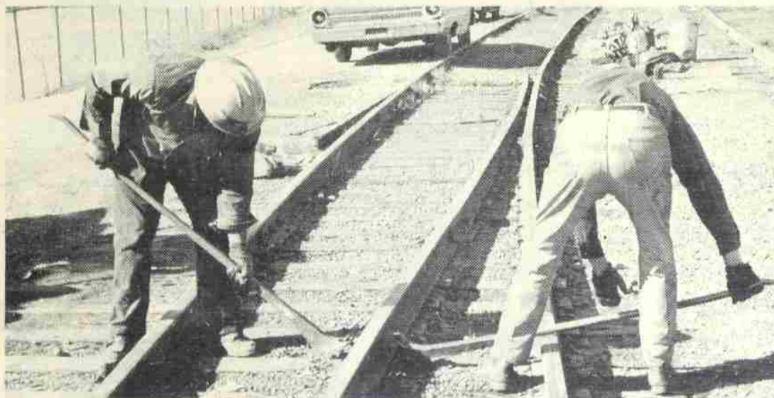
It's a good start Southern Pacific! However it appears the removal of this switch which served the former Salem Navy warehouse is the only reduction in trackage for the campus. Among colleges, Willamette shares the distinction of being bisected by Southern Pacific rails with institutions such as OSU in Corvallis. The best WU can hope for is a few landscaping improvements if Southern Pacific's plans remain static.
