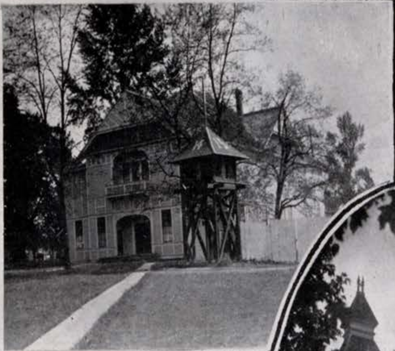
Gym and Bell Tower
