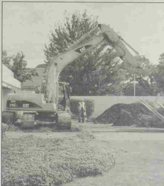
Construction recently began on the new Kaneko Commons.
