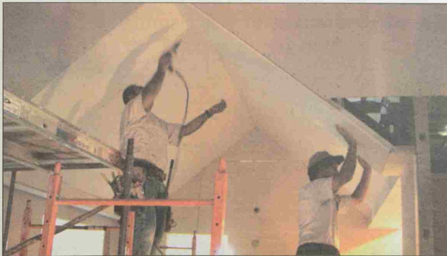
A pair of workers install the new roof and rafters in the fourth floor of Eaton Hall.
