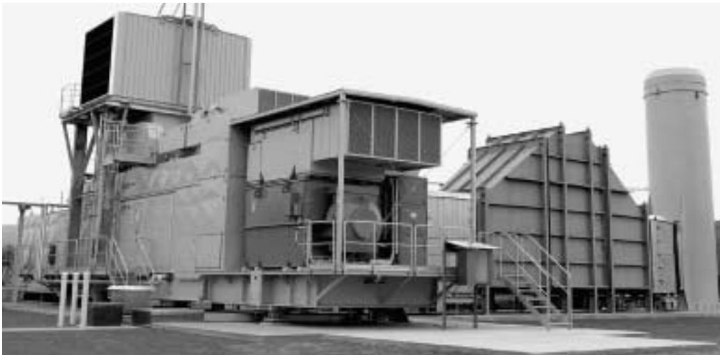
The 24.5 MW simple cycle gas turbine (which does not include a steam turbine) was planned by PGE in response to the regional energy crunch last winter and was brought on line within six months of conception. Known as a 'peaking resource' it can be started and stopped quickly typically between the hours of 6 a.m. to 10 a.m. and 4 p.m. to 8 p.m. weekdays. The plant can power about 20,000 homes under normal
