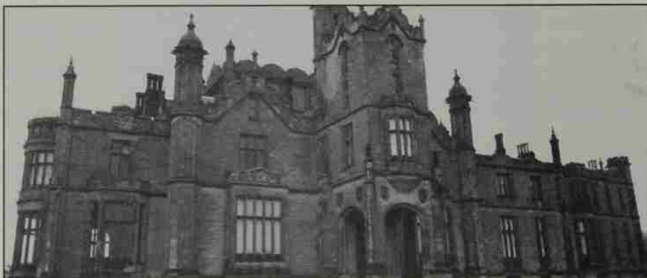
More than an acre of slate roof covers this Victorian country house in England. Once owned for a time by the Duke of York, Allerton has been described in Landscape Magazine as "not really a country house but rather the House of Lords transported to the Yorkshire countryside."
