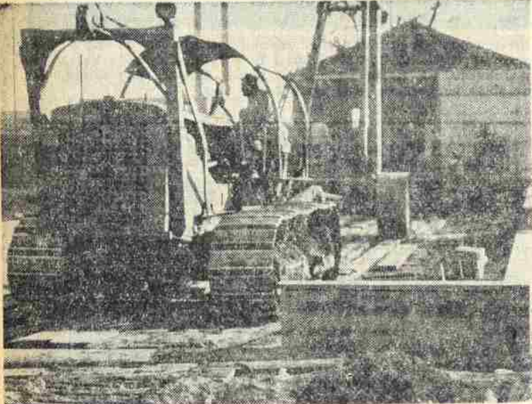
Bulldozers clear ground in the initial stages of Baxter hall construction.
