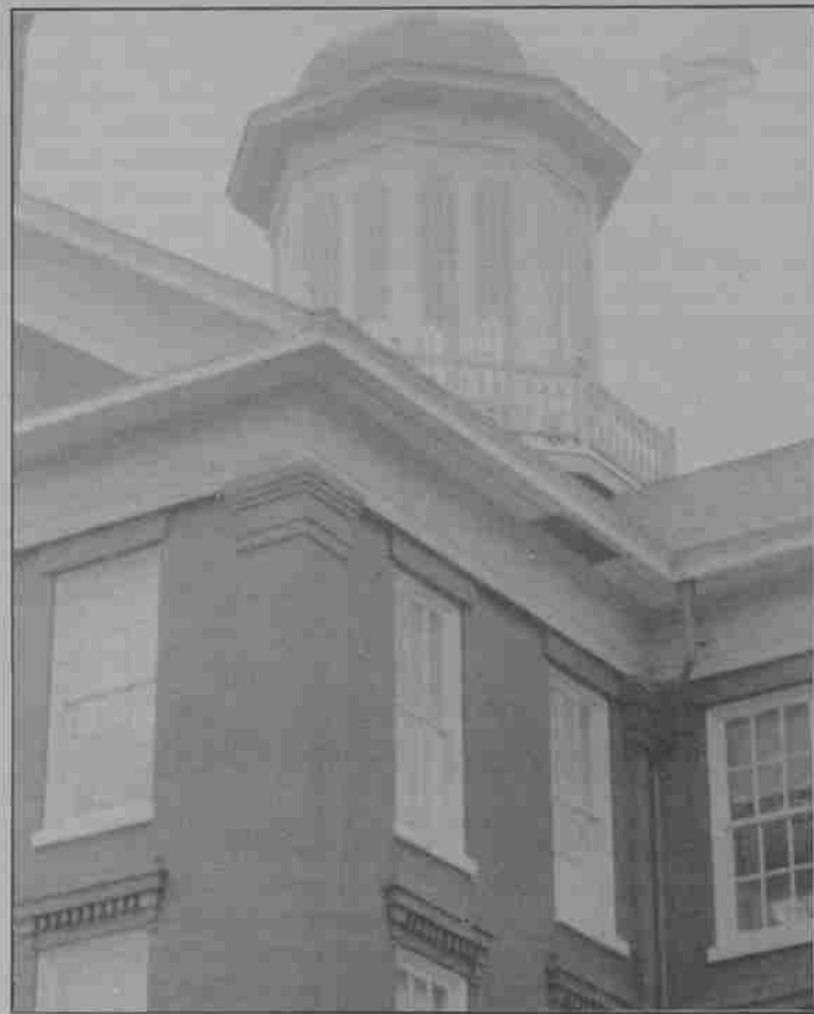
Cone Chapel, located in Waller Hall, might become the center of an Oregon branch of the Methodist Theological School in Ohio, reviving a seminary tradition began with the Kimball School of Theology, which closed in 1930.
