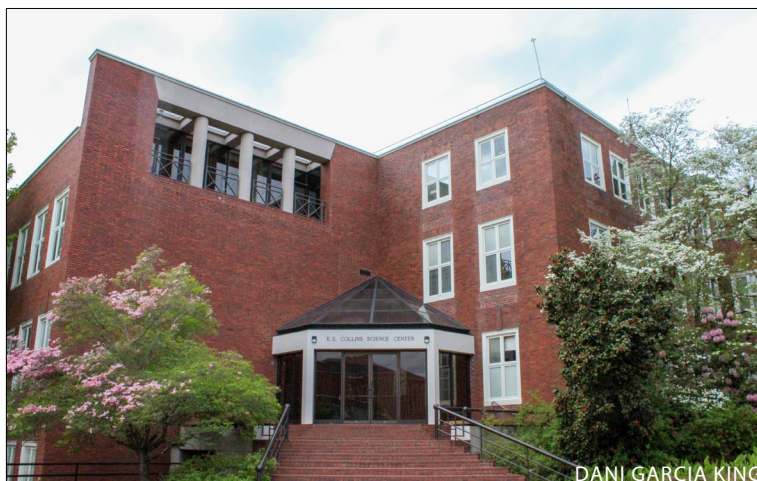
Colins, which houses many of Willamette's science departments, now closed.
