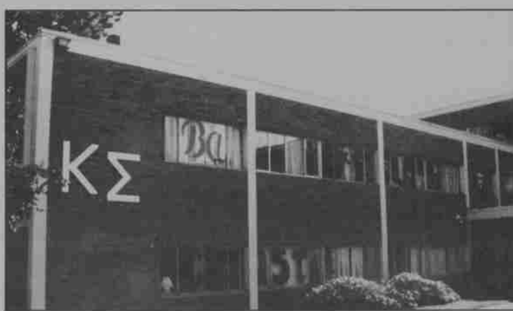
Kappa Sigma is working with Robin Smithro of the Office of Disability Services to renovate their house to make it more accessible to Ryan Skelton, a disabled Kappa Sigma member.
