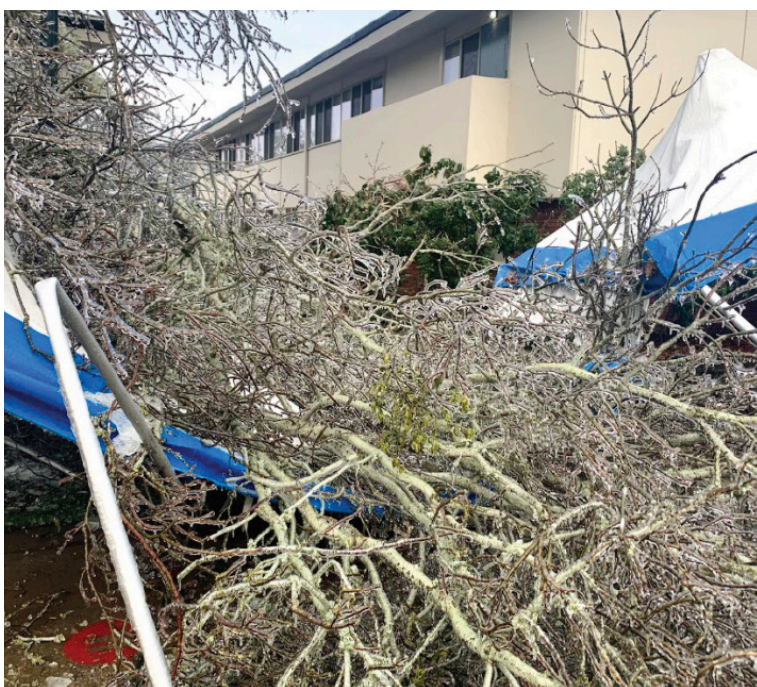
Branches fell and crushed tents covering the waiting area for Goudy Commons.
