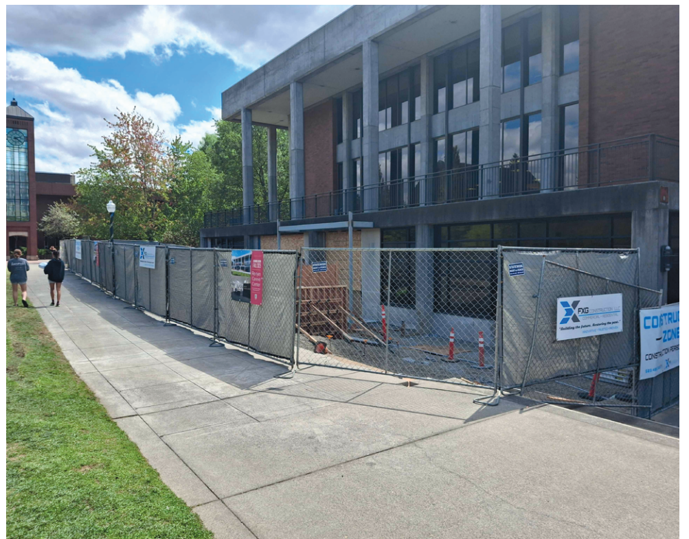
Construction of the new Renjen Career Center on Aug. 18, 2025.
