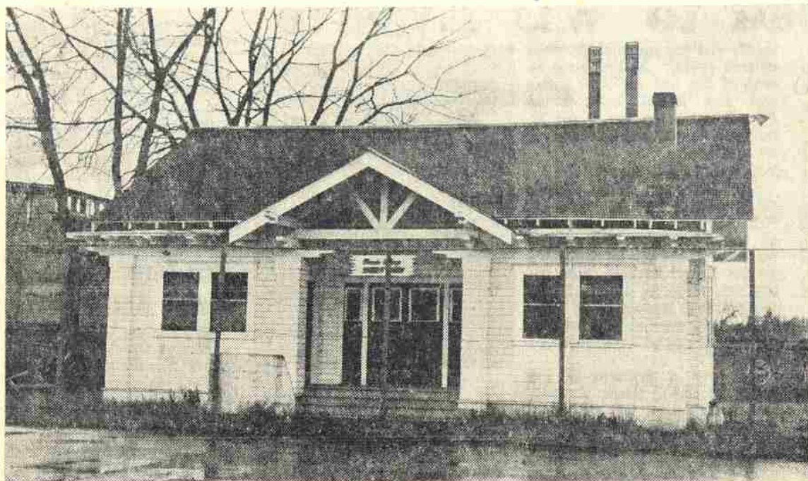
Chresto cottage, the student union of 1918, has had a long history of varied service to Willamette university. It witnessed a revolution in social customs as well as a number of moves. The pair of chimneys which seemingly pierce the roof is not part of a new heating unit but stacks from some unknown cannery.
